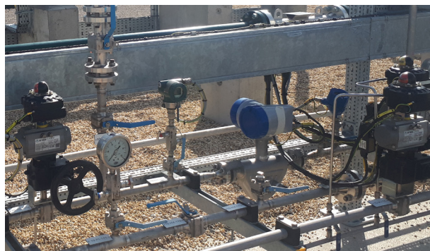
Flow measurement of hydrogen and SNG with the OPTIMASS 6400
