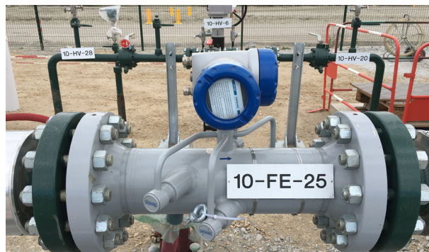
OPTISONIC 7300 ultrasonic flowmeter prior to commissioning
