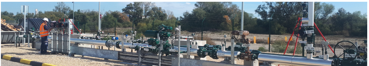
OPTISONIC 7300 C: Ultrasonic flow measurement of natural gas from the grid
