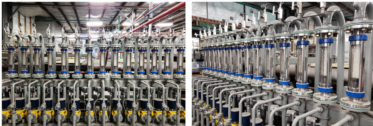
Hydrogen flow measurement with the VA 40 variable area flowmeter
